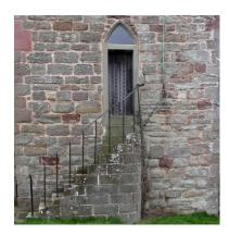
The lower window on the west wall of the tower has been enlarged and converted to a doorway to the bellringers' chamber. The stone steps leading to the door and the iron handrail were installed soon after November 1845, when Sir Samuel Meyrick wrote to a friend about it. Access to the floors inside is by ladder. A steep ascent leads to the bell chamber itself from the ringers' chamber. A full description of the bells can be found in the Heritage Trail for inside the church.
